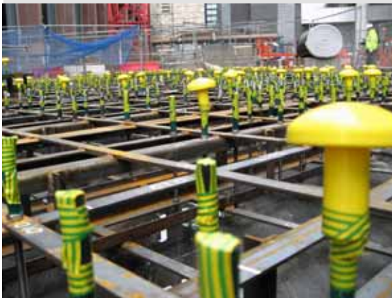
Figure 6: Bolt cage prior to concrete pour
