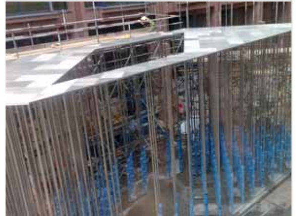
Figure 8: Pavilion under construction
